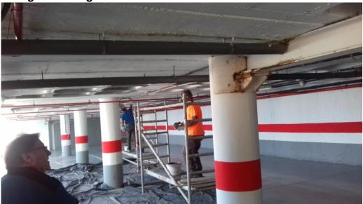
The ceiling in the garage area on 10th floor has had leakages, and small pieces concrete have fallen down. The areas in question have been sealed.
